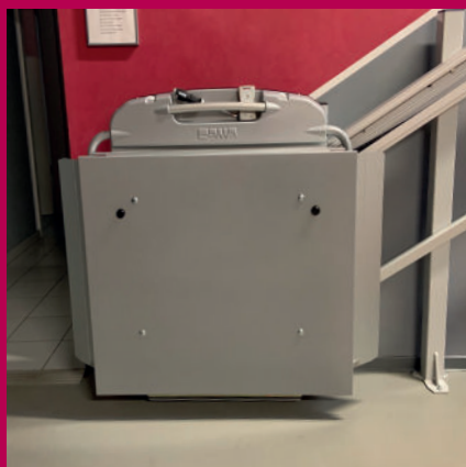
Platformslift lige trappe
